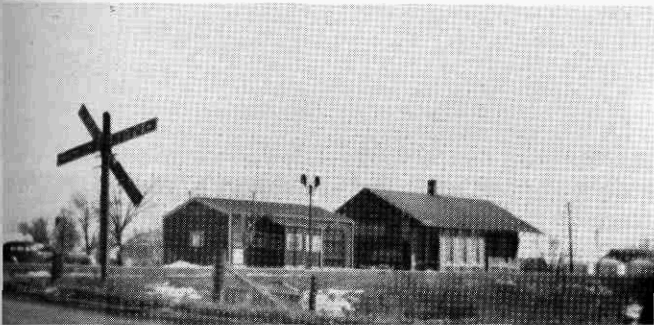
The new and the old. Semaphore-type train order signal has given way to new flashing light system. Soon the old depot will be dismantled and removed.
