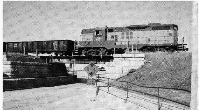
CNW work train picks up the pieces in 1982.
