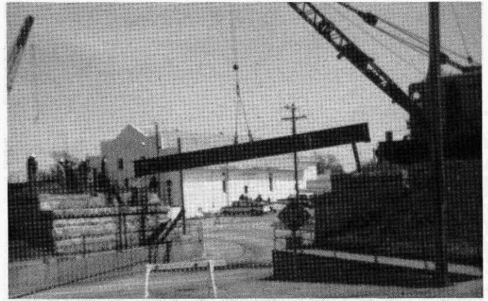
The last beam of the viaduct is removed, April 1982.
