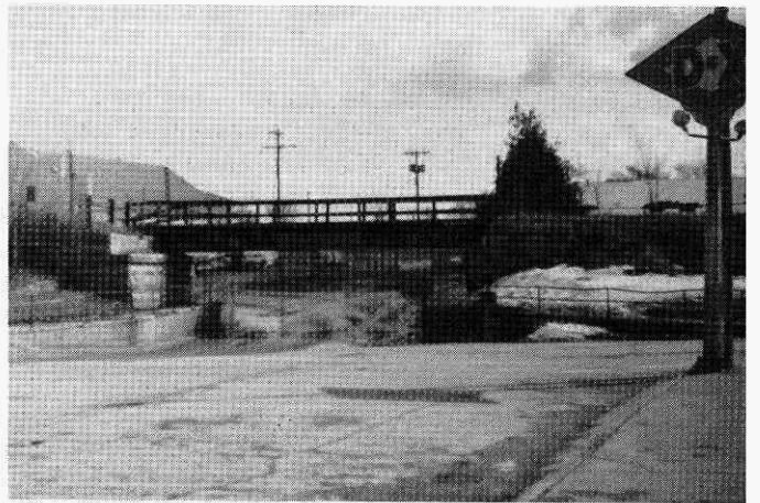
Looking east to the viaduct.
