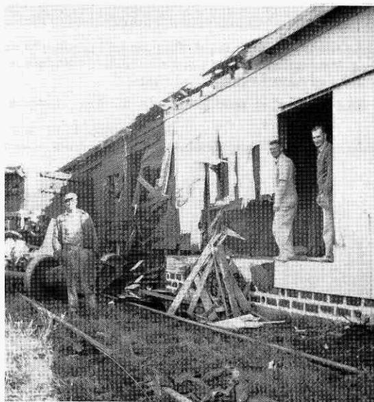
Cars derailed next to the Eclipse Lumber Company warehouse in 1951.
